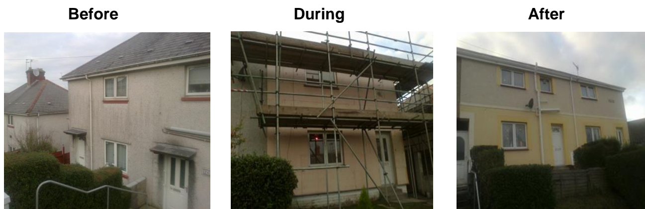
Figure 3 – Typical Enveloping Scheme 1
